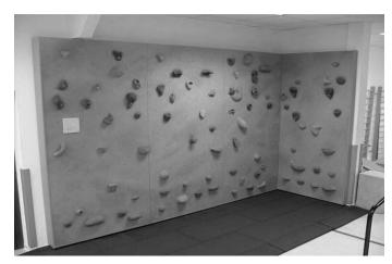
**Figure 1.** A therapeutic climbing wall. The total lateral length is 4 m and the height is 2.5 m. The wall is equipped with duroplastic holds of different sizes, shapes, and colors.
